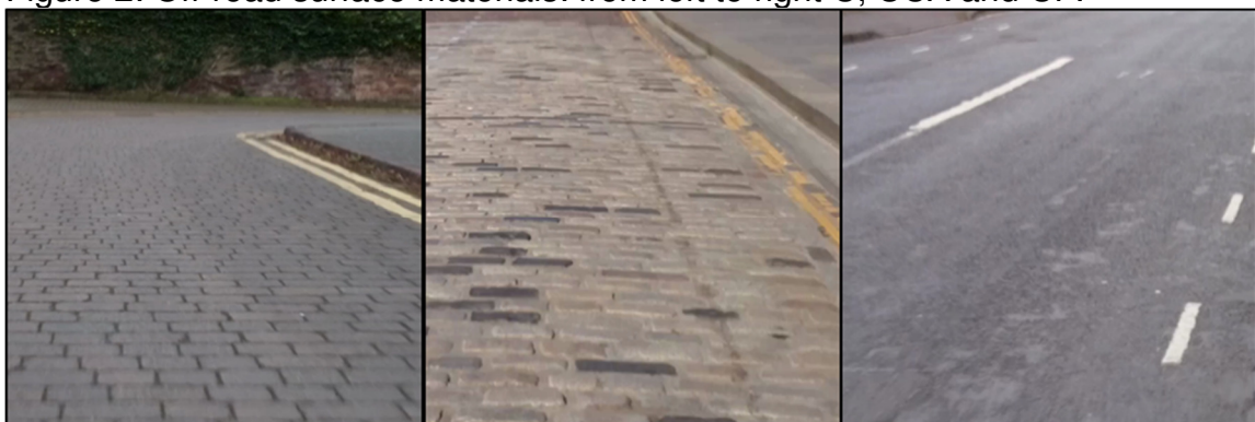
Figure 3: Road pavement surface materials: from left to right CB, CS and HRA.
