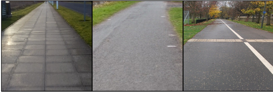
Figure 1: Off-road pavement surface materials: from left to right CP, AC and HRA.
