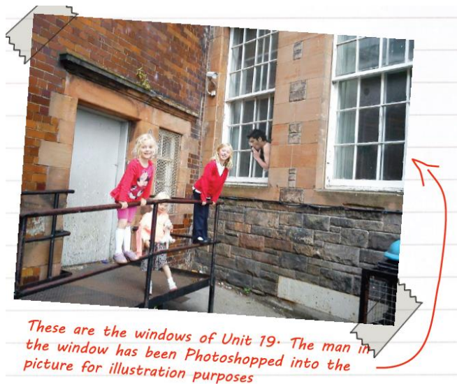
Figure 42: Photo of Ground Floor Window with Smoker Added
