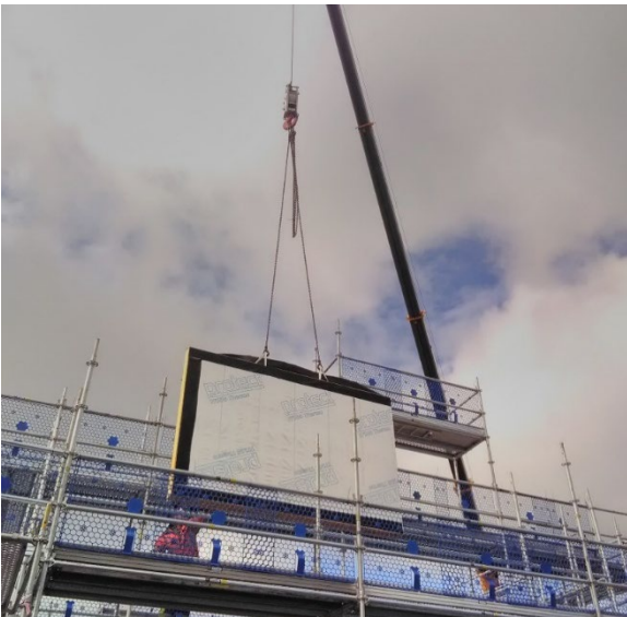
Figure 6 Wall panel being lifted into position
