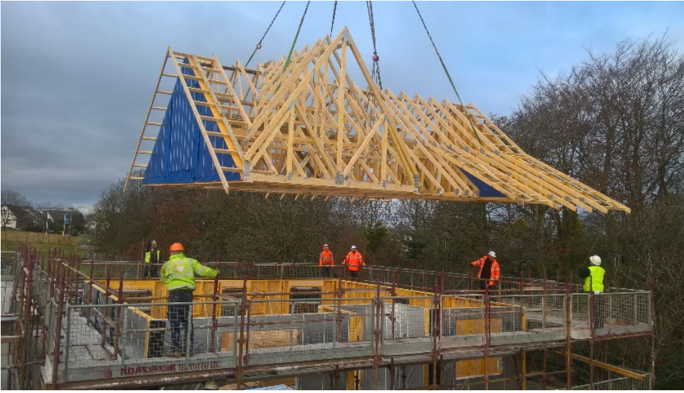
Figure 5 Roof trusses being lifted into position as one piece
