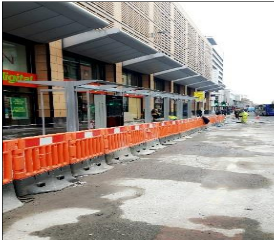
Figure 7.6: Fastlink halt during construction (Source: Author's image)
