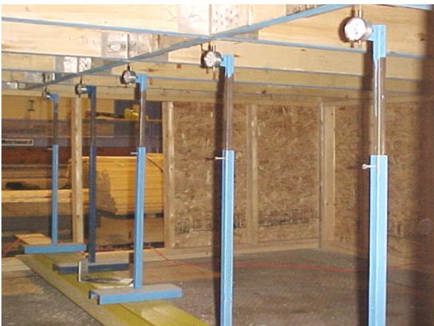
Figure 10: Dial gauges for measuring mid-span deflections of joists
