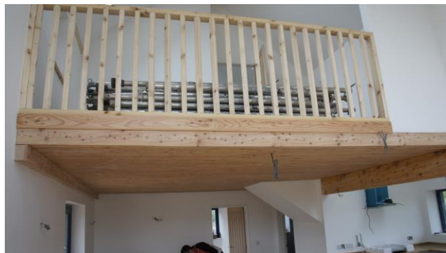
Figure 5 - Dowel-lam intermediate floor in practice
